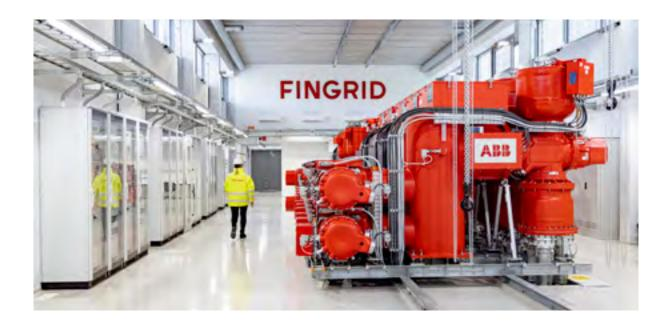
When connecting to a gas-insulated Fingrid switchyard by cable coming outside of the fenced switchyard area, the ownership and management of the lines at the switchyard end at the Connecting Party's cable and the cable-side connectors of the cable terminations in Fingrid's GIS switchgear output. The connectors on the side of the circuit breaker bay's cable terminal of the switchgear in question are owned by Fingrid.
