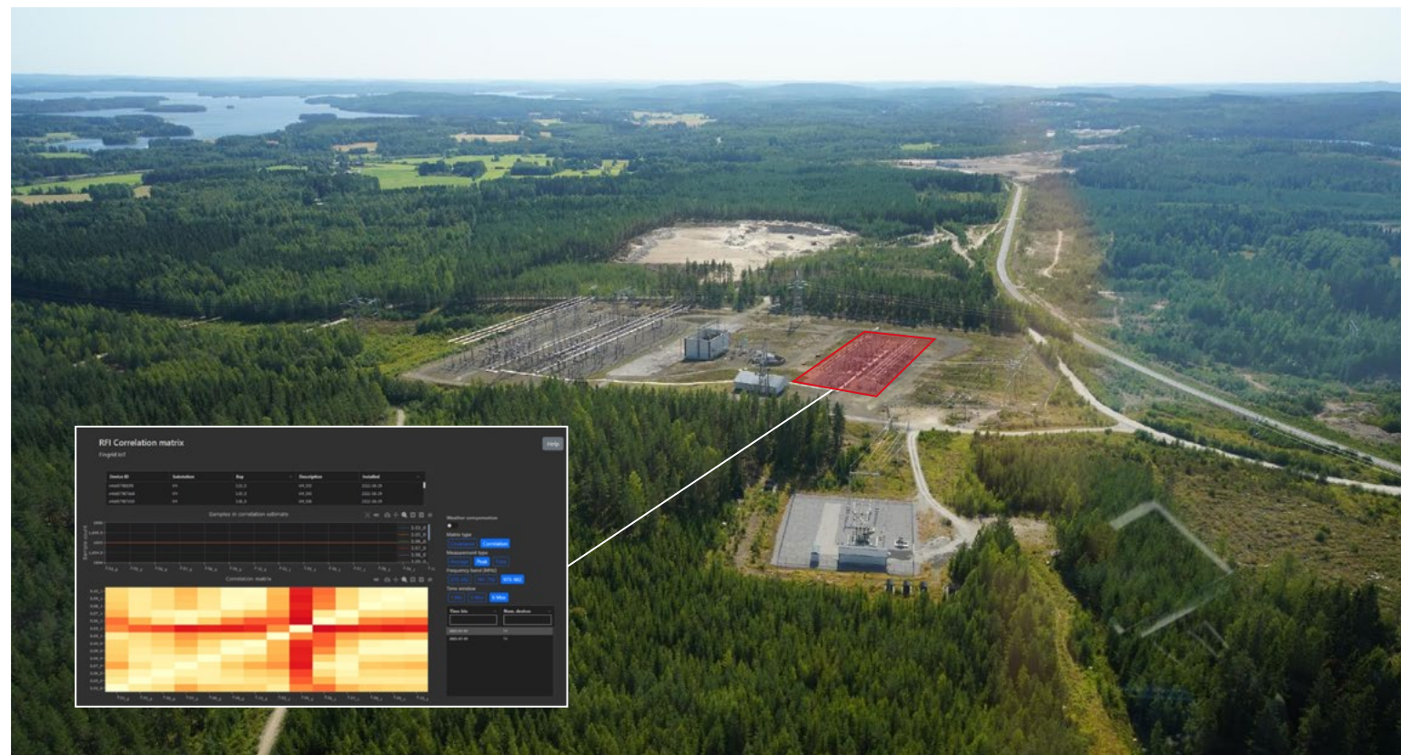
Figure 35. Digital condition management systems can detect deviations in substation equipment. Pictured: the Vihtavuori substation in Laukaa.
