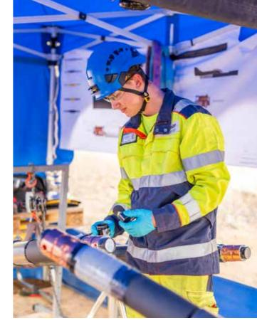
Additional earthing is an important safety measure. It can ensure that a work location in a high-voltage installation is unenergised and eliminate hazardous induced voltages in work locations.
