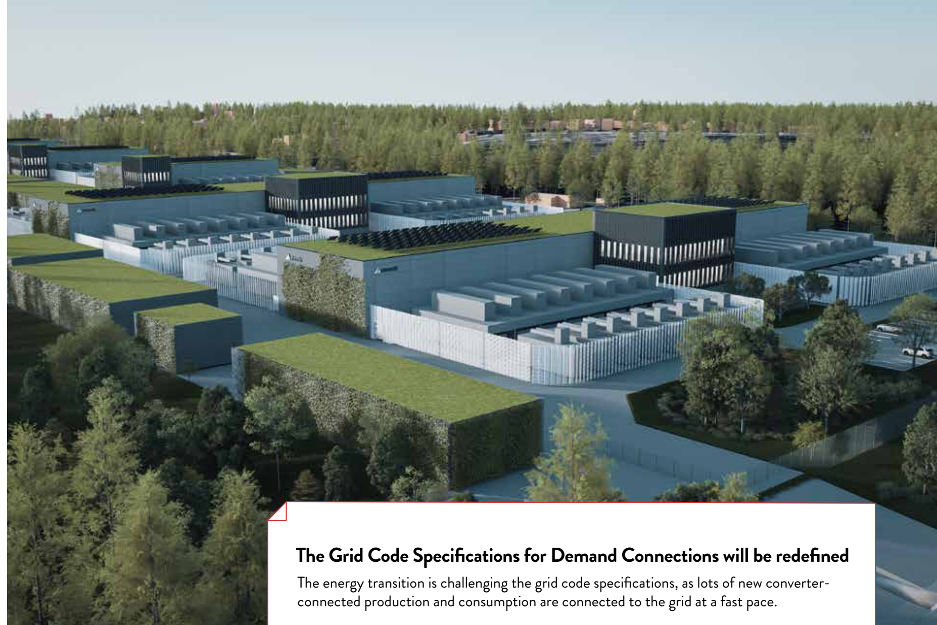
atNorth is building a data centre in Myllykoski, Kouvola, which will ultimately have a capacity of several hundred megawatts. Illustration.
