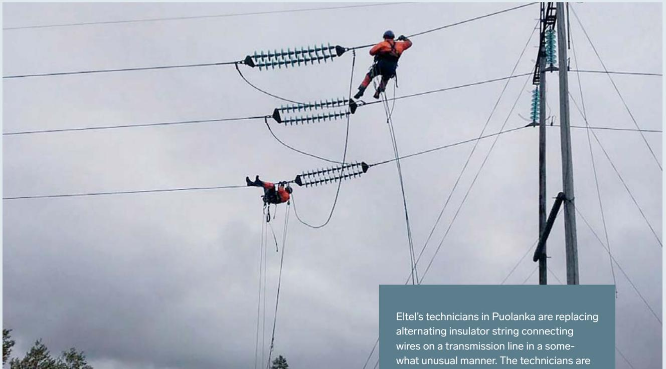
Eltel's technicians in Puolanka are replacing alternating insulator string connecting wires on a transmission line in a somewhat unusual manner. The technicians are attached to the conductor with harnesses and suspension seats and they are using lowering ropes and lift handles.
