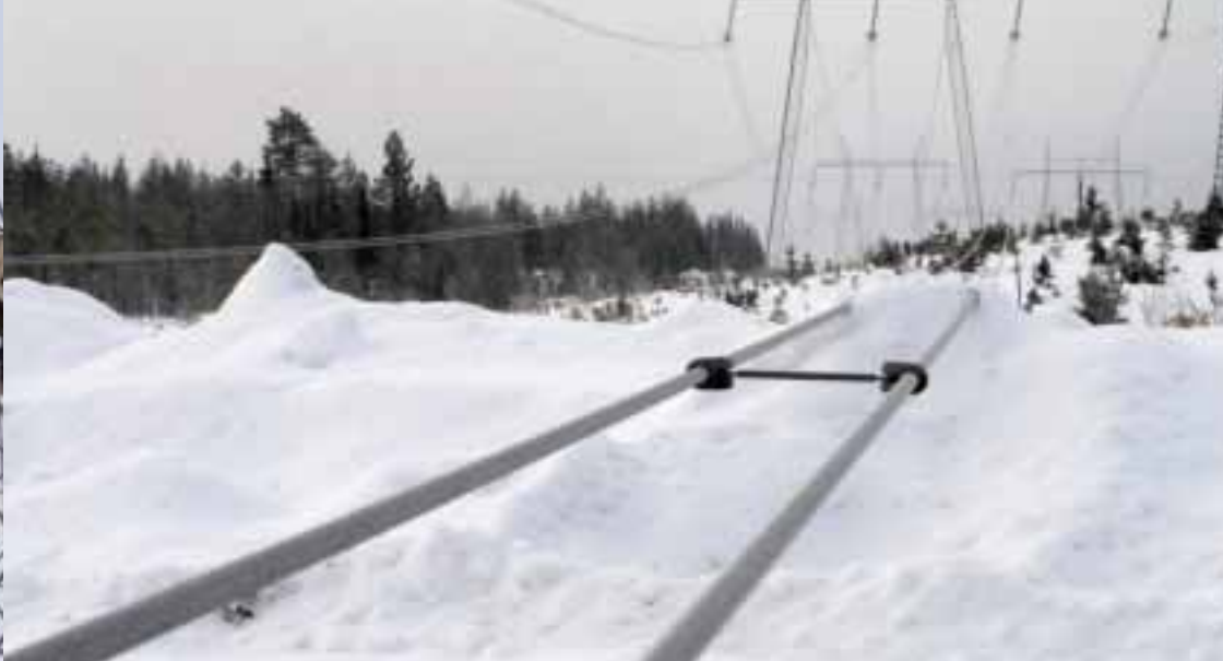
The current conductors (3 x 2 Finch) were not replaced. Only worn or damaged conductor accessories were replaced.
