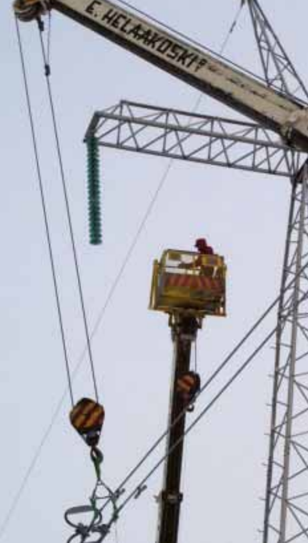
The current conductors (3 x 2 Finch) were not replaced. Only worn or damaged conductor accessories were replaced.
