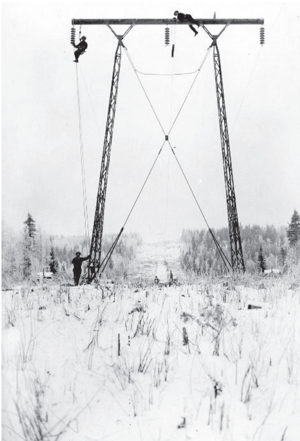
The safety equipment used when working on transmission line towers has developed a lot since the time this photo was taken in the 1930s.
