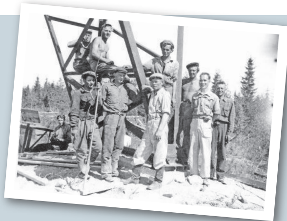
Foreman Laakso's hoisting group at the base of the Haapajärvi crossover tower in summer 1948.
