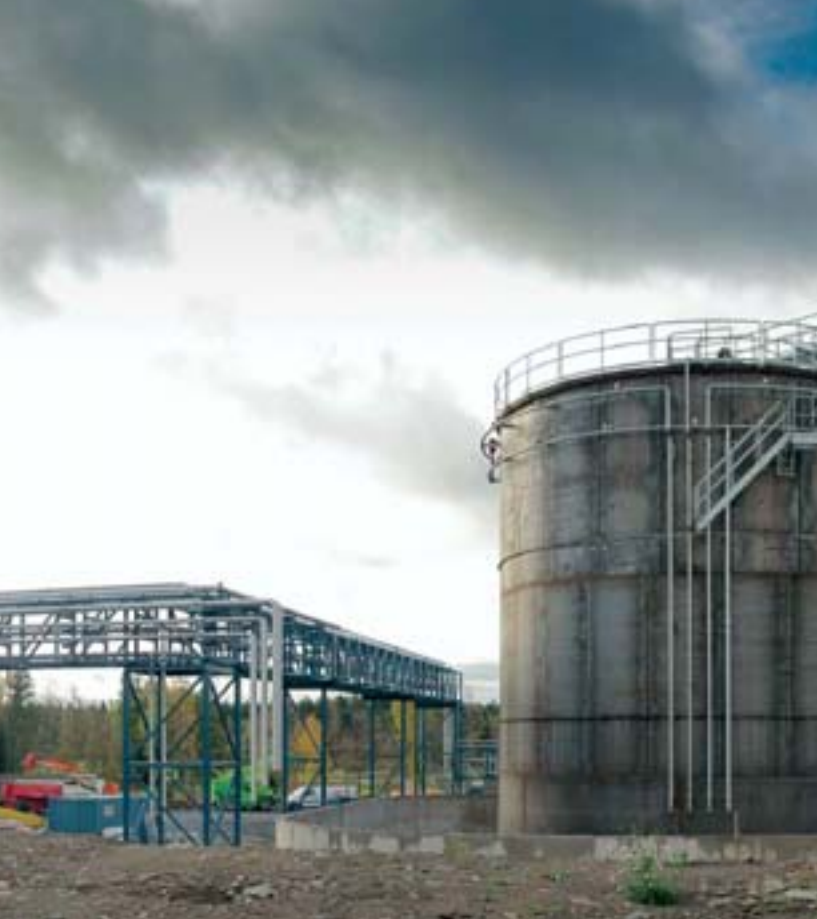
Construction work for the Forssa reserve power plant was largely completed in 2011. The 300 megawatt gas turbine plant is due to be ready in the autumn of 2012.
