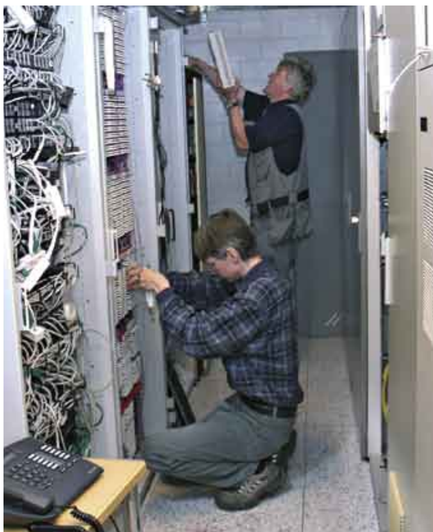
Lauri Puskala and Pentti Ahlqvist dismantling the old telephone network.
