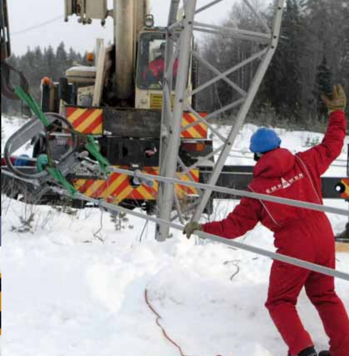
The conductors are lowered before the aluminium tower is turned over.
