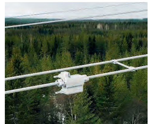
The sensor analyses the sag of the cable and monitors the swaying caused by the wind.
